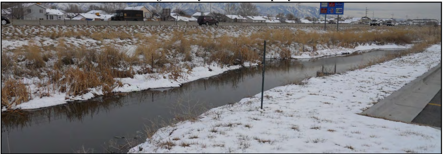
Current Condition of Detention Basin
